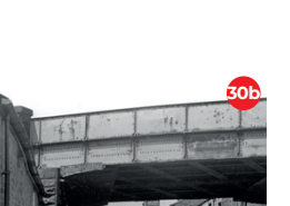
The railway bridge crossing over School Lane, Brinscall
