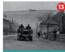
Salt Pie House visible on the right of the car.
