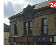
No. 2 Co-operative Society Branch Bury Lane, Withnell Mill
